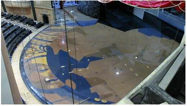
andling Specialty custom engineered, manufactured and installed one of the world's first and largest underwater stage systems for Cirque du Soleil's groundbreaking Las Vegas show, "O". The show takes place in a pool containing 1.5 million gallons of water. Four hydraulically-actuated lifts raise and lower the four-piece stage which measures 3,650 square feet.
