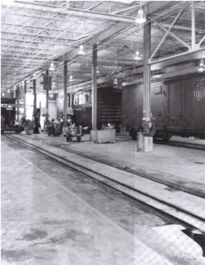
Progression of cars through shop workstations is a popular ROBOT application. Enclosure of puller ropes is added safety factor.
